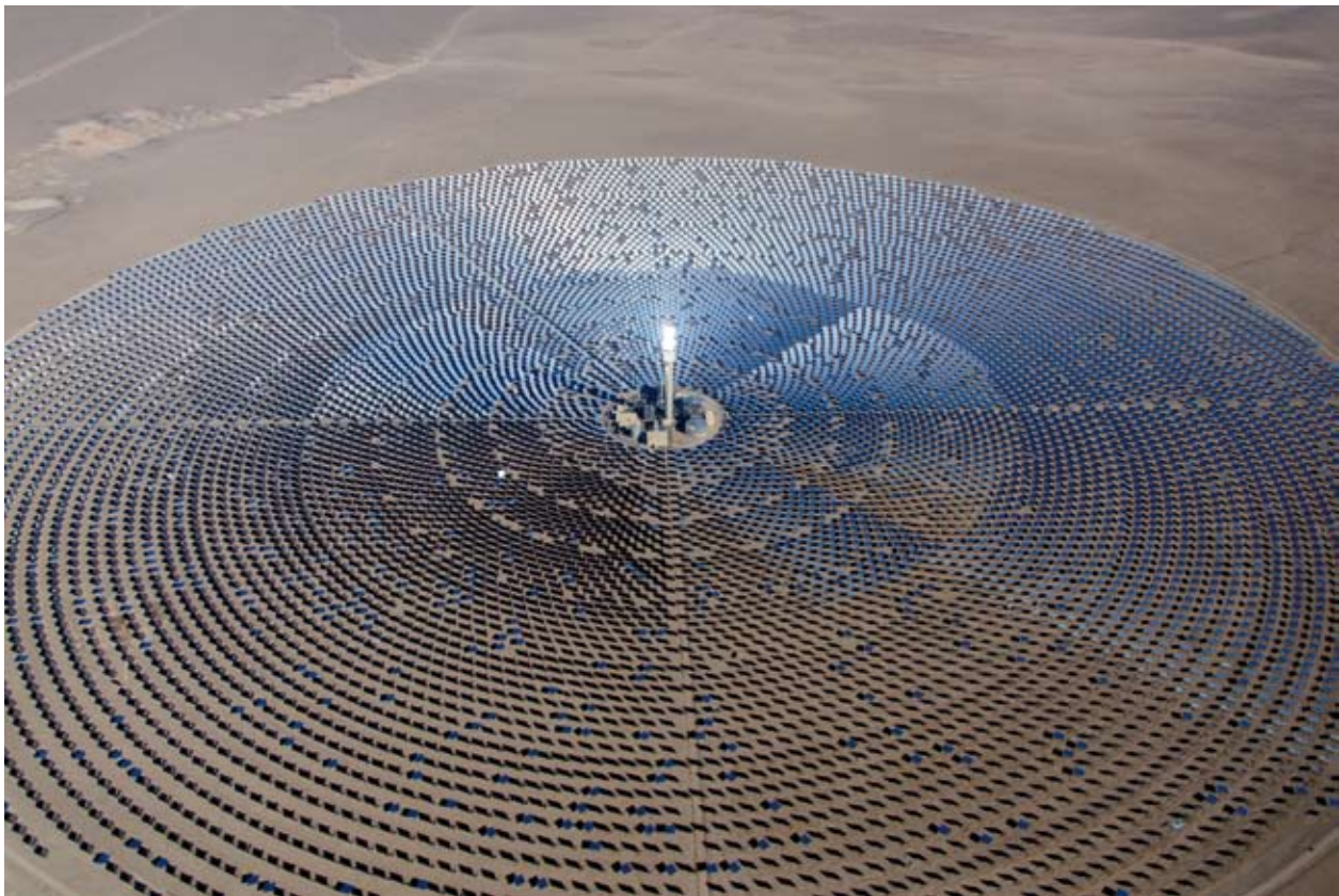
The Crescent Dunes Solar Thermal Energy project in Nevada. The 2.6 square miles of mirrors reflect and concentrate the sun's rays onto the receiver in the center, heating the molten salt it contains. When electricity is needed, the stored heat is used to generate steam and power a turbine, just like a traditional power plant. Photo: U.S. Bureau of Land Management via Flickr, CC BY 2.0.
